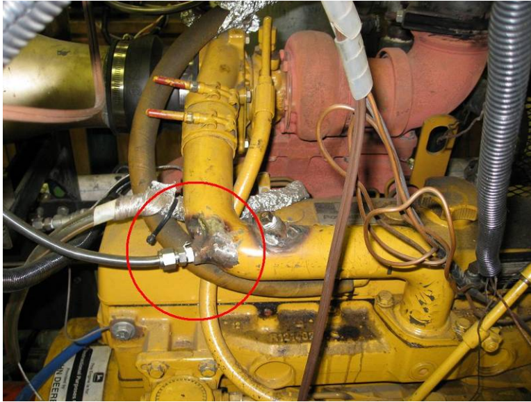
Figure 1 – Ammonia intake location.
